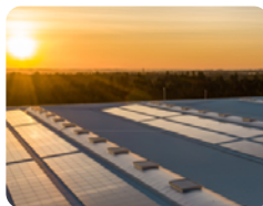
Solar Powered Warehouse Panels
