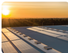
Solar Powered Warehouse Panels
